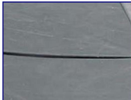
*Often, the sections of modular parks do not sit flush or line up correctly, causing an extreme skating hazard.*
