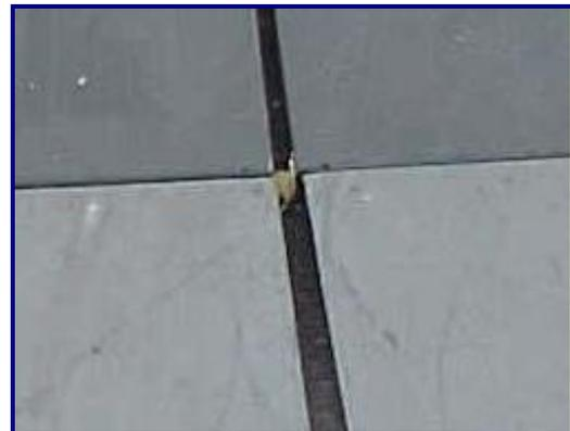
*Thresholds that are separated and lifted off the ground present a danger to users of improperly constructed skateparks.*
